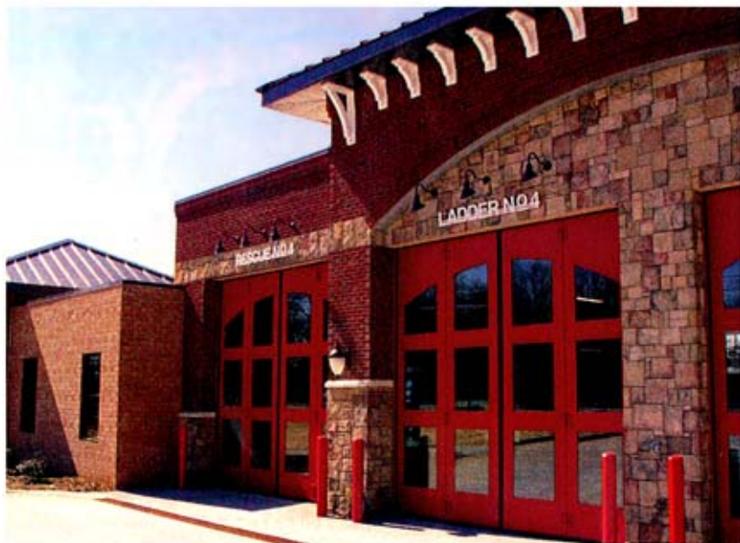
These state-of-the-art bifold doors are a first for a fire station in North Carolina. Operated by a flywheel, control arms and a 5-horsepower motor, these doors take five seconds to open, can operate half a million cycles before requiring maintenance, and, in the event of a power failure, can be opened by one man in less than 30 seconds.
